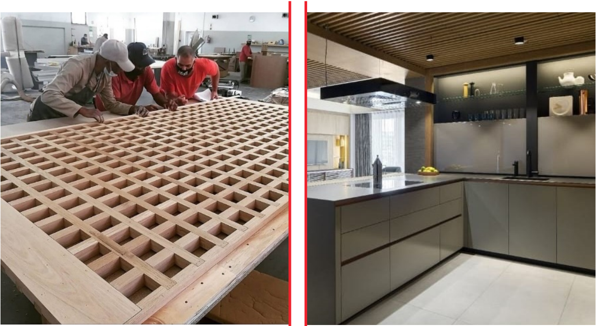
Figure 11: Kitchen ceiling deck during production and after installation
